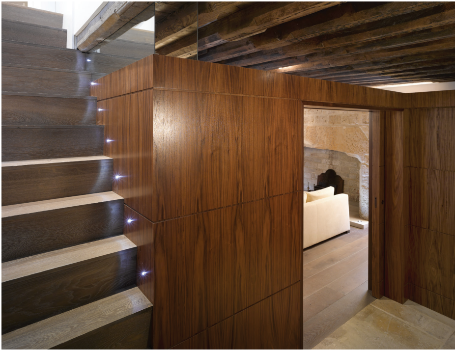
The long lifetime of LED lightbulbs makes them ideal for fitted lighting structures such as this staircase
